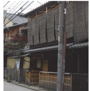
Figure 13. The facade of g5 having cascade glazing with cross lines
